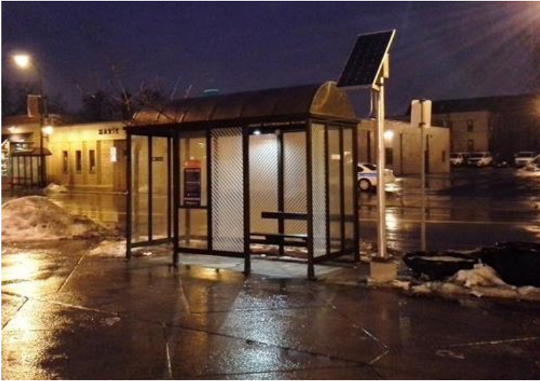
Figure 14 Metro Transit Solar Powered Bus Stop
